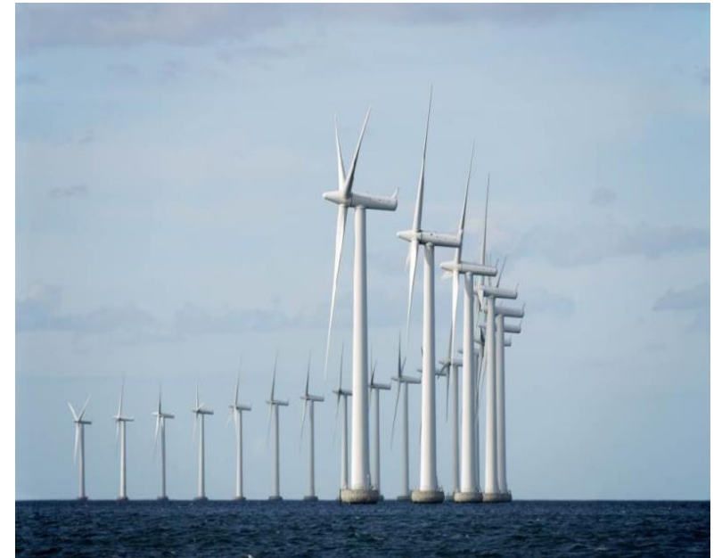
Middelgrunden, Denmark. Source: R&D A/S, retrieved from https://www.offshorewind.biz/2020/12/23/denmarks-iconic-offshore-wind-farm-to-get-a-new-lease-on-life/
